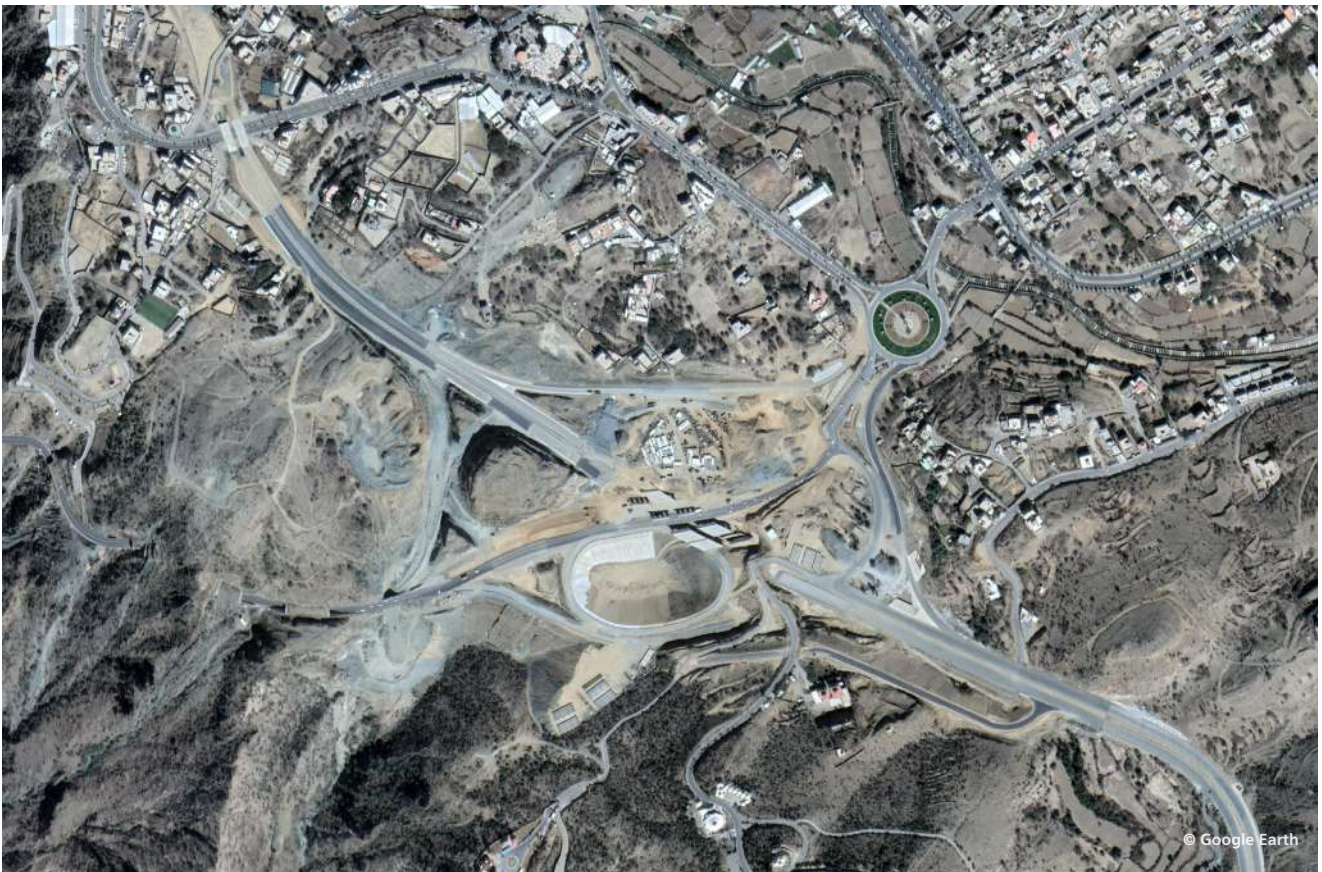
Overdimensioned and cost intensive interventions like the construction of the intersection of the new Ring Road
