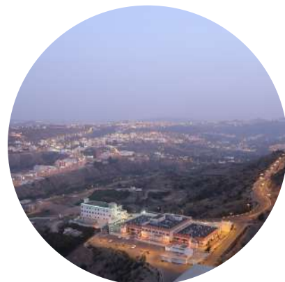
Disconnected and inaccessible major public infrastructure such as the main hospital disrupt the functionality of the city
