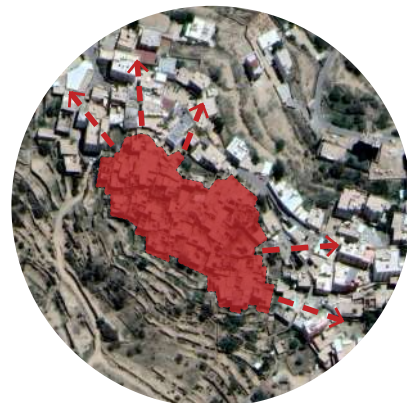
Building activities are taking place around the vernacular structure.
