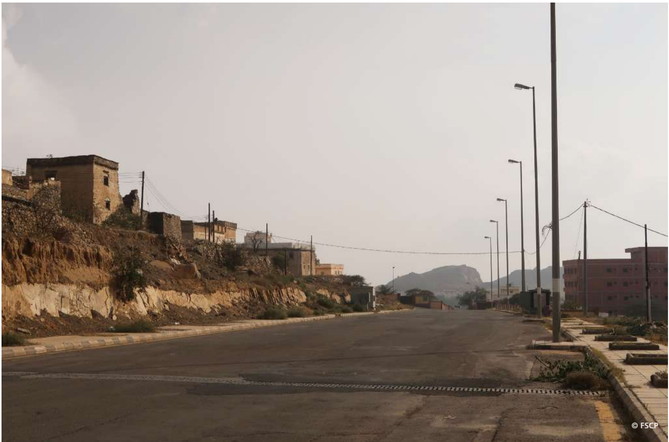
Oversized and pedestrian unfriendly road design in the city centre
