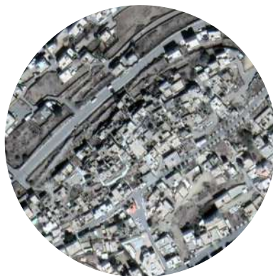
2. Partly overbuilt vernacular structure
