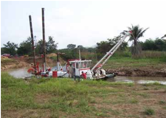
Figure 7-22 . Dredging of the Densu River Channel at Nsawam
