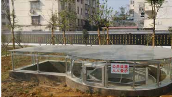
Figure 4-9 First application of large-scale hydrodynamic vortex separator for wet-weather overflows in China
