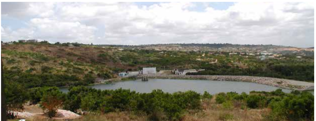
Figure 7-19 Section of the Weija Dam and Reservoir
