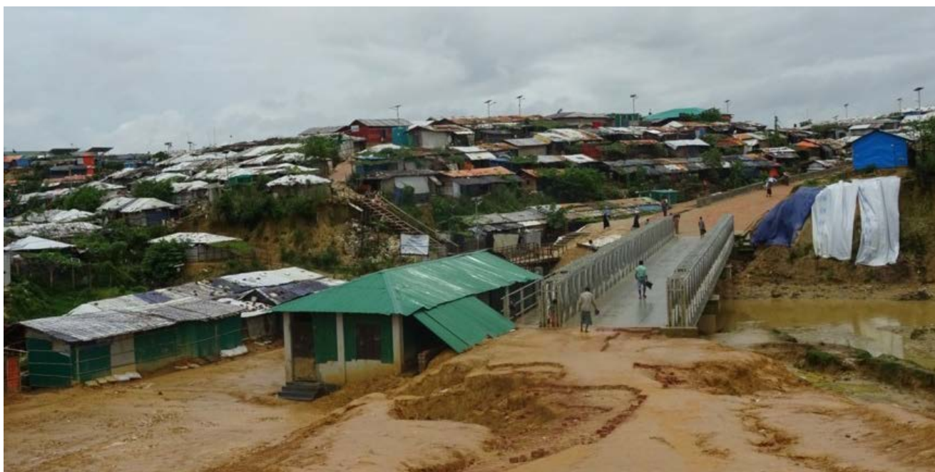
An example of rapidly constructed settlements created without long-term urban planning in Cox's Bazar, Bangladesh © UN-Habitat
