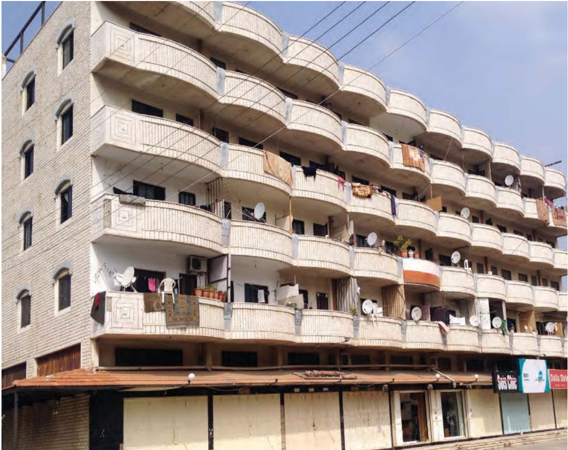
Picture 12: Apartment complex - Akkar , Lebanon
