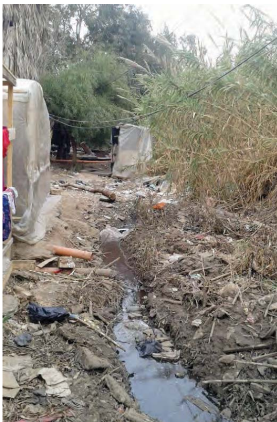
Picture 2: Improvised water drainage and sewage channel in an ITS - Akkar, Lebanon
