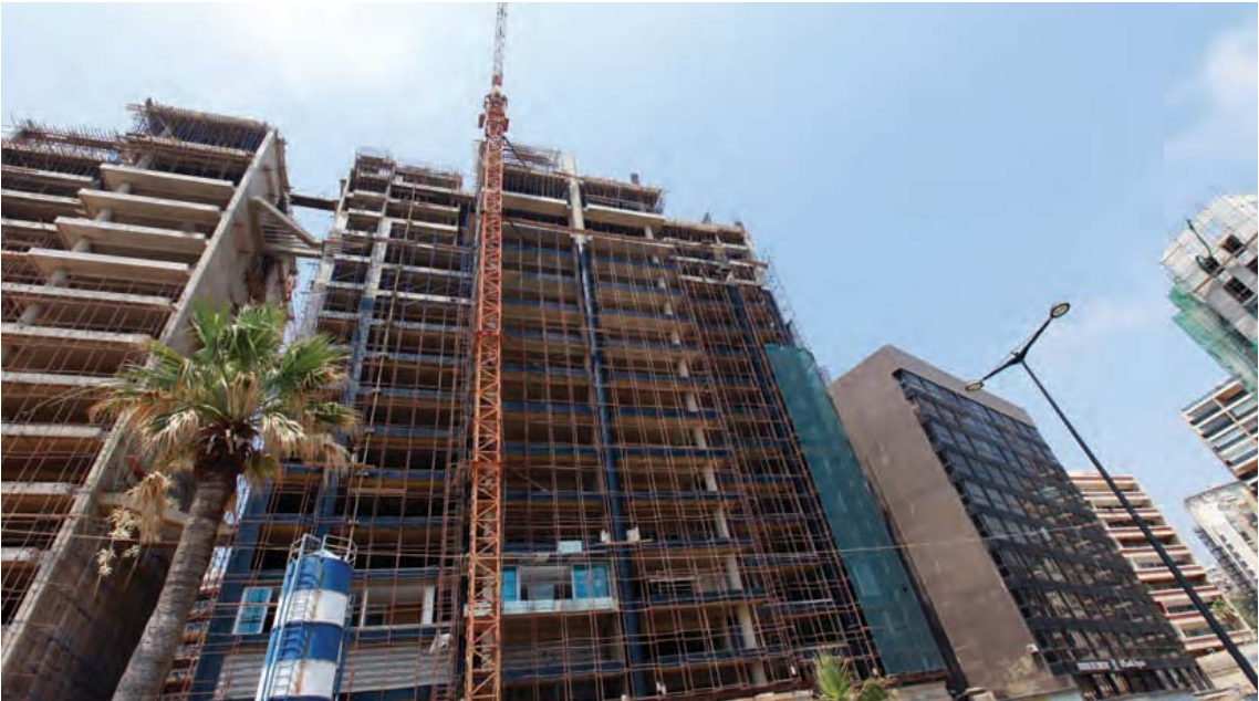
Picture 4: Building under construction - Beirut, Lebanon
