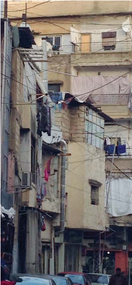
Picture 6: Vertical additional unit in Naba'a - Beirut, Lebanon
