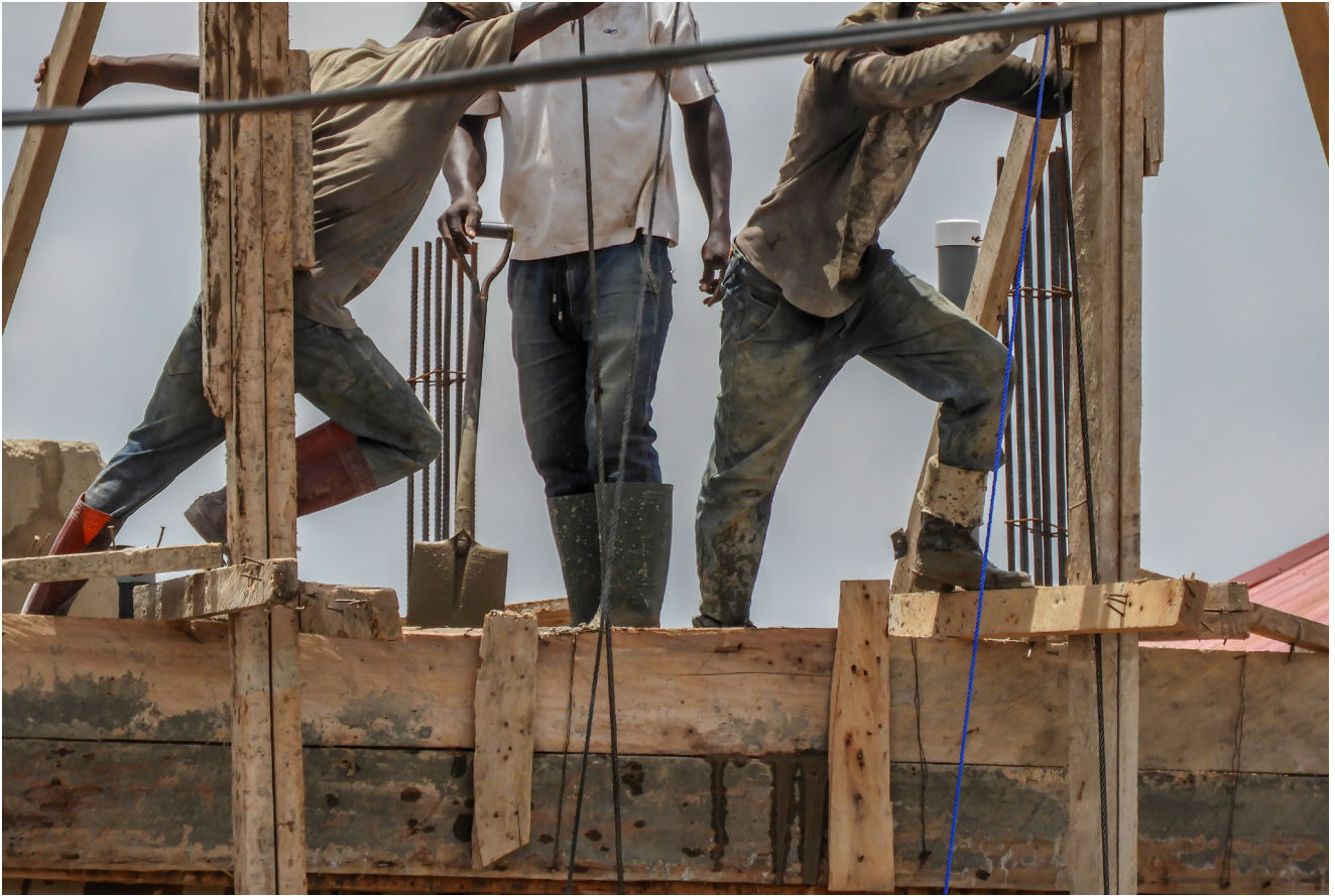
Workers building houses in Accra city, Ghana © SHUTTERSTOCK/Gerhard Pettersson
