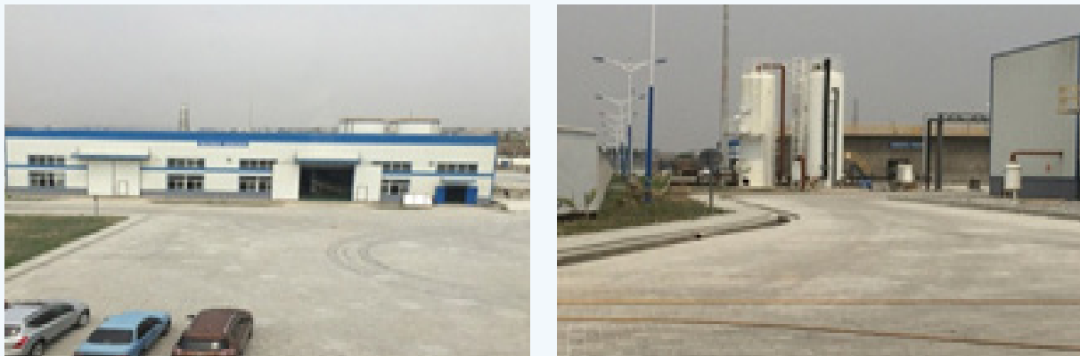
Figure 2.7 Septage Treatment Plant in Accra
