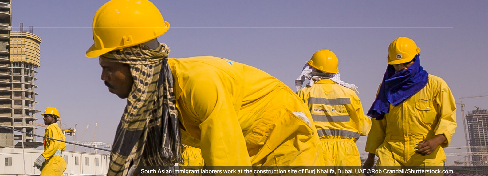
South Asian immigrant laborers work at the construction site of Burj Khalifa, Dubai, UAE ©Rob Crandall/Shutterstock.com
