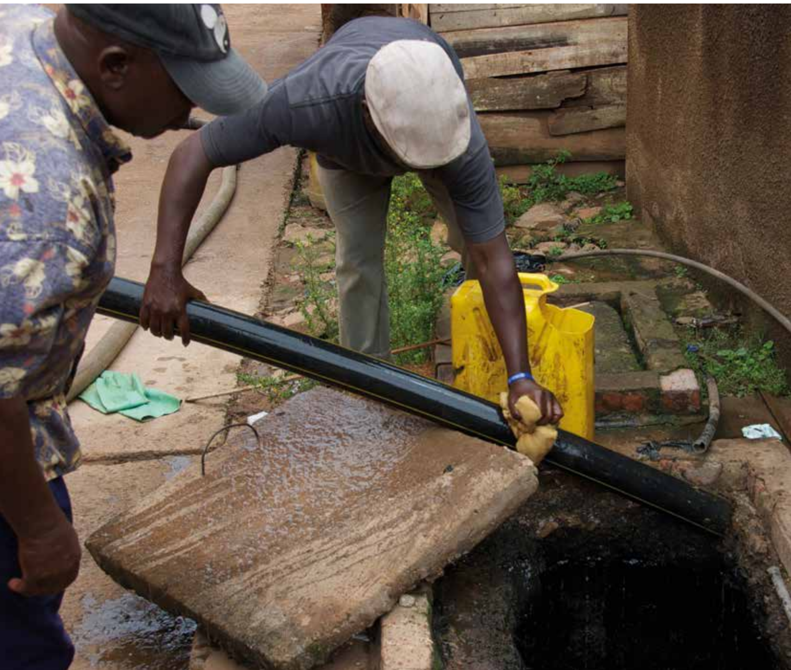
Pipe cleaning in Kampala, Uganda. Photo: Lars Schoebitz
