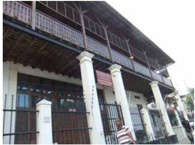
FIGURE 3.11-27 THE HIGH COURT OF TANZANIA, DAR ES SALAAM: VIEW FROM THE STREET, PORTICO AND GALLERY SHADED TO REDUCE SOLAR GAINS
