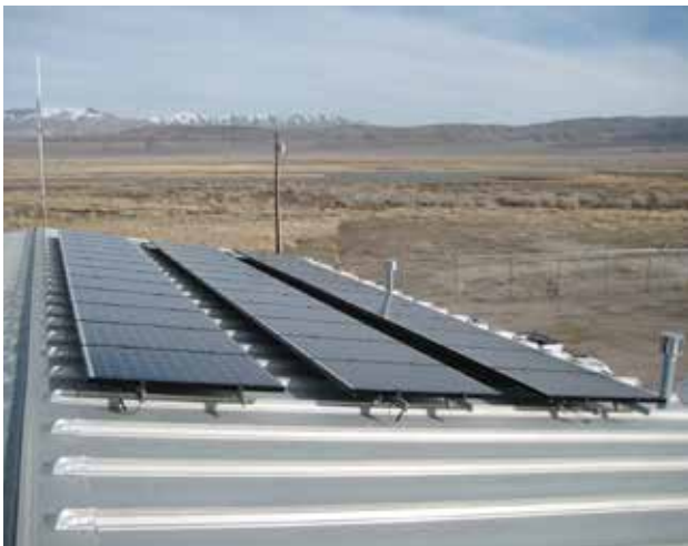
FIGURE 6.1-3 PV ON PITCHED ROOF
