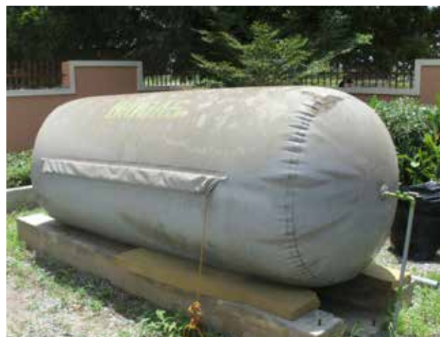
FIGURE 6.4-16 ABOVE GROUND PLASTIC INFLATABLE GASHOLDER
