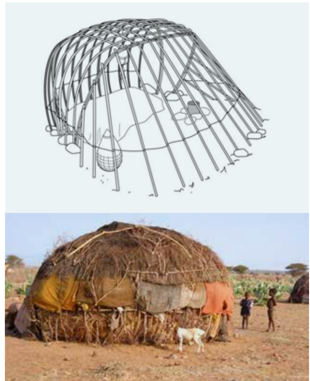
FIGURE 3.11-5 WOODEN STRUCTURE AND REAR SIDE OF THE MIN COVERED WITH THATCH
