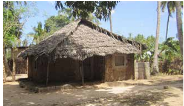
FIGURE 3.11-17 SWAHILI TRADITIONAL HOUSE IN KIGAMBONI (DAR ES SALAAM, TANZANIA)
