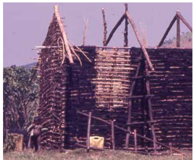
FIGURE 3.11-15 MUD BONDED WITH STICKS AND REEDS APPLIED TO A FRAME MADE OF WOOD
