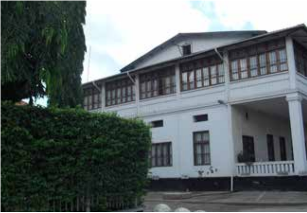
FIGURE 3.11-26 LARGE OPENINGS AND VERANDAS FOR NATURAL VENTILATION
