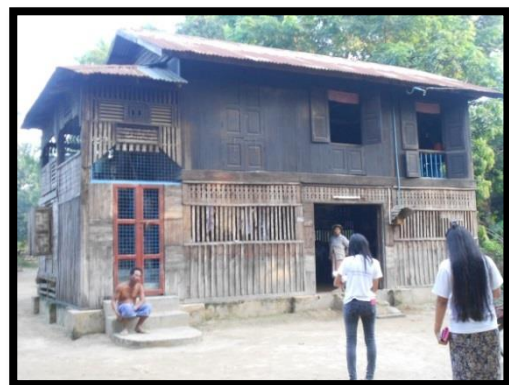
Timber Building (W1L)
