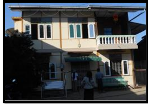
Brick Nogging Building (RM1L)
