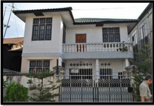
Reinforced Concrete Building (C3L)
