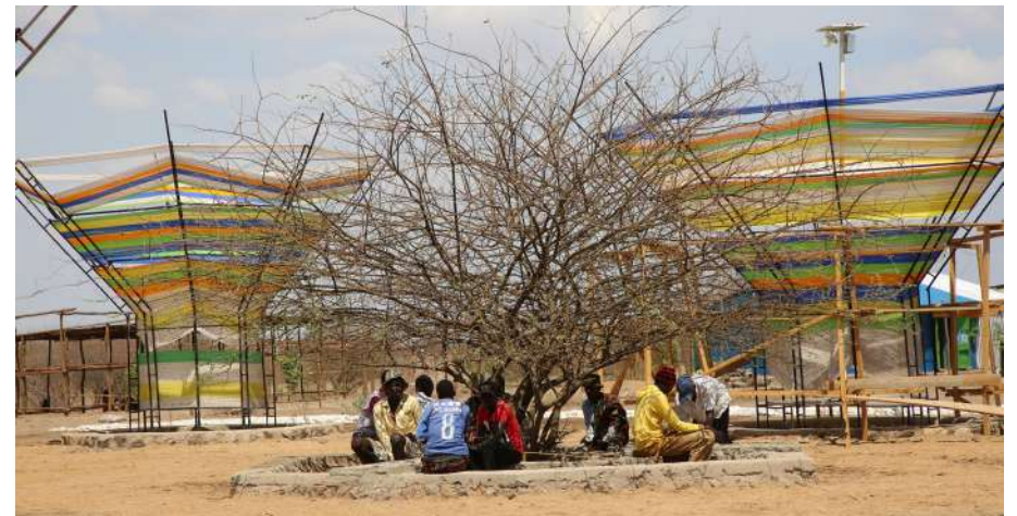
Completed installation of artificial shading structures
