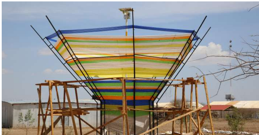
A solar lamp is installed in the middle of the shading structure to provide for lighting at night
