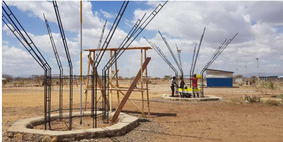
Metal structures for shade are erected on the site
