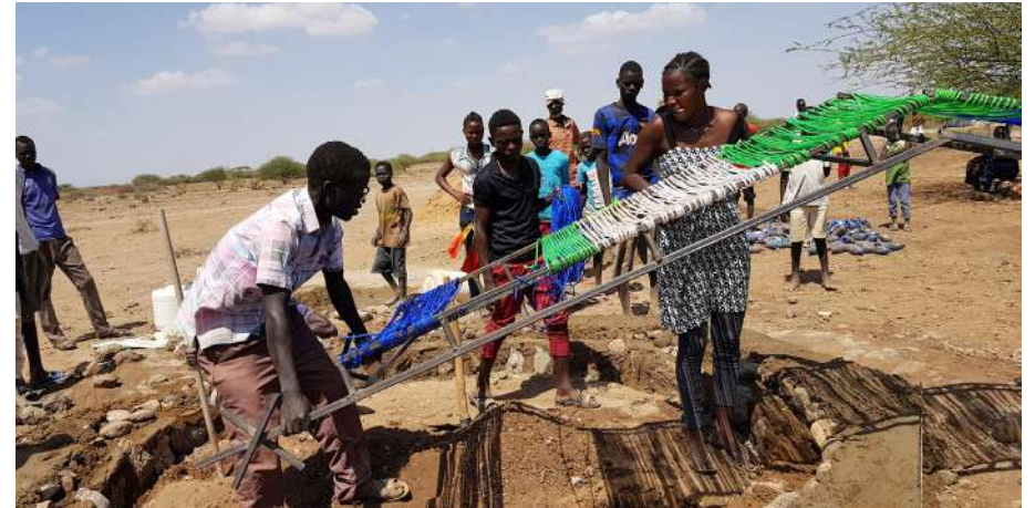
Community members work together to raise the weaved shade structure onto site
