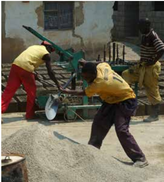
Construction in Zambia © UN-Habitat
