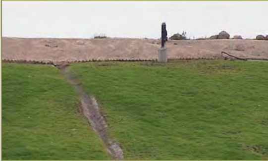
Gas venting pipe on waste dump
