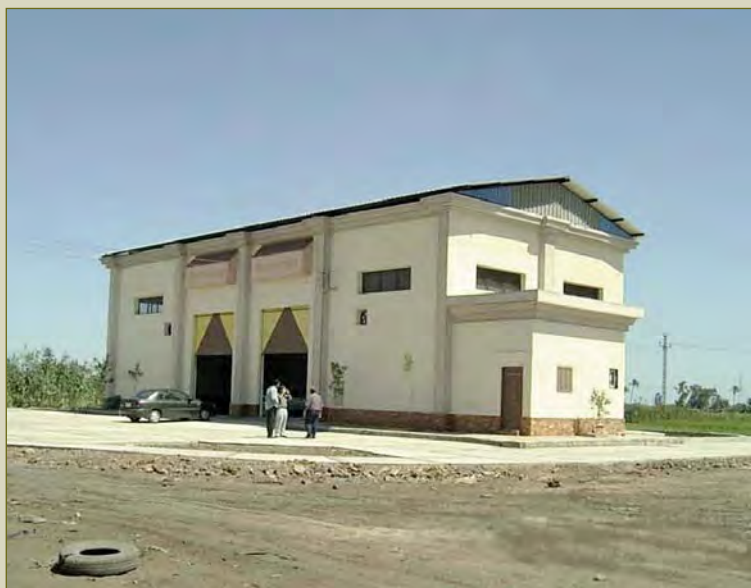
Transfer station at Faraskour, Egypt. The design is suitable for up to 150 tonnes/day capacity
