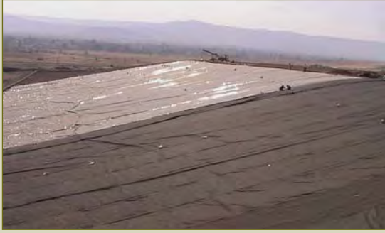
Laying HDPE liner
