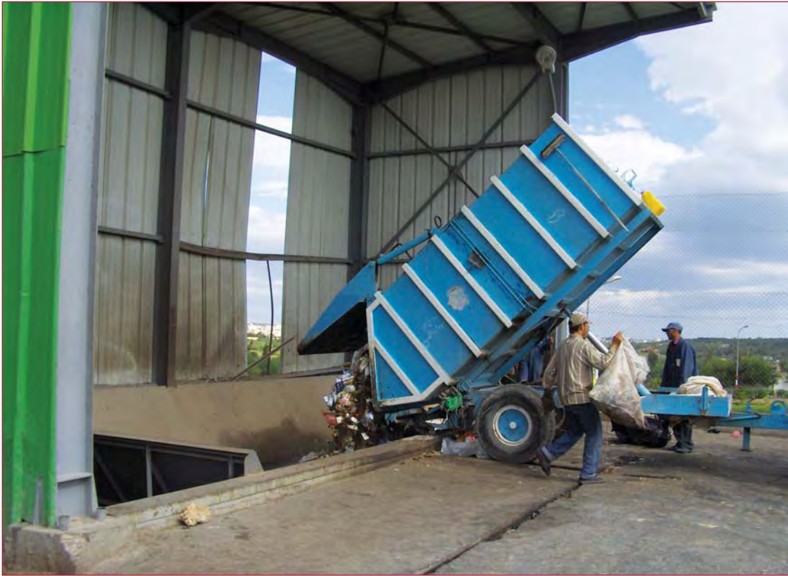
Transfer station in Sousse, Tunisia
