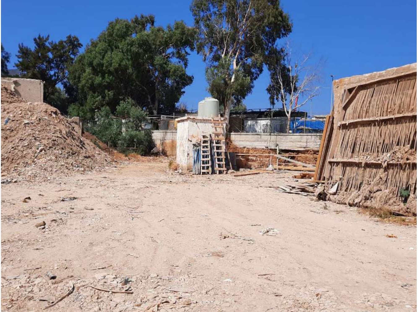
On-Site Fixed Structure, Bakalian Waste Storage Site / UN-Habitat © 2021
