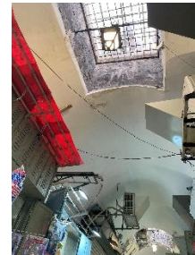
Photos No.: 4 Skylight at Khan El-Zeit-Photo credit: Evaluator
