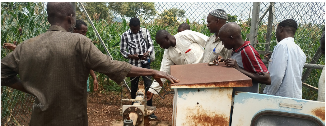
» Technicians doing repair work on the Tegina Bi-Water Scheme
