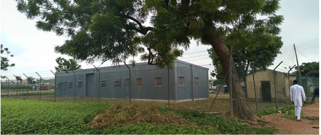
» Rehabilitated Gwada Bi-Water Scheme
