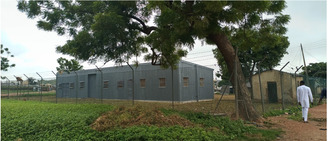
» Rehabilitated Gwada Bi-Water Scheme
