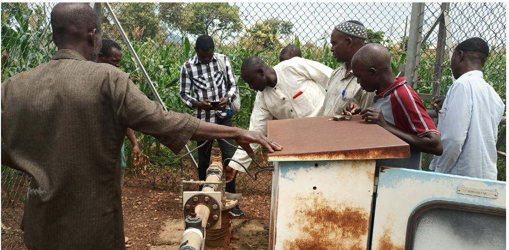
» Technicians doing repair work on the Tegina Bi-Water Scheme
