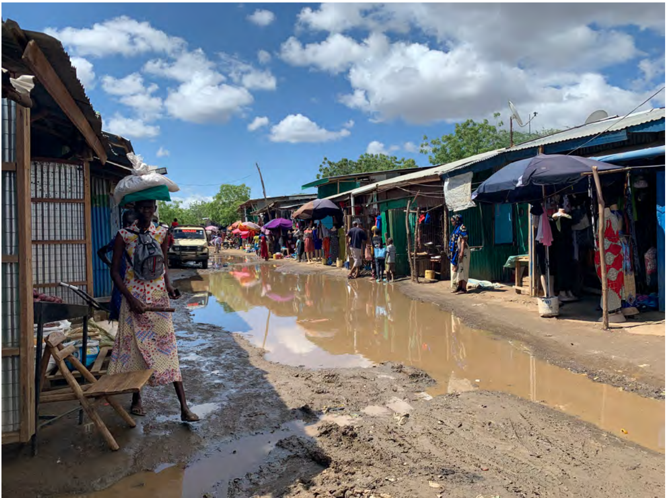
Fig. 32: Flooded Section of Ethiopian Market Street (UN-Habitat, 2022)
