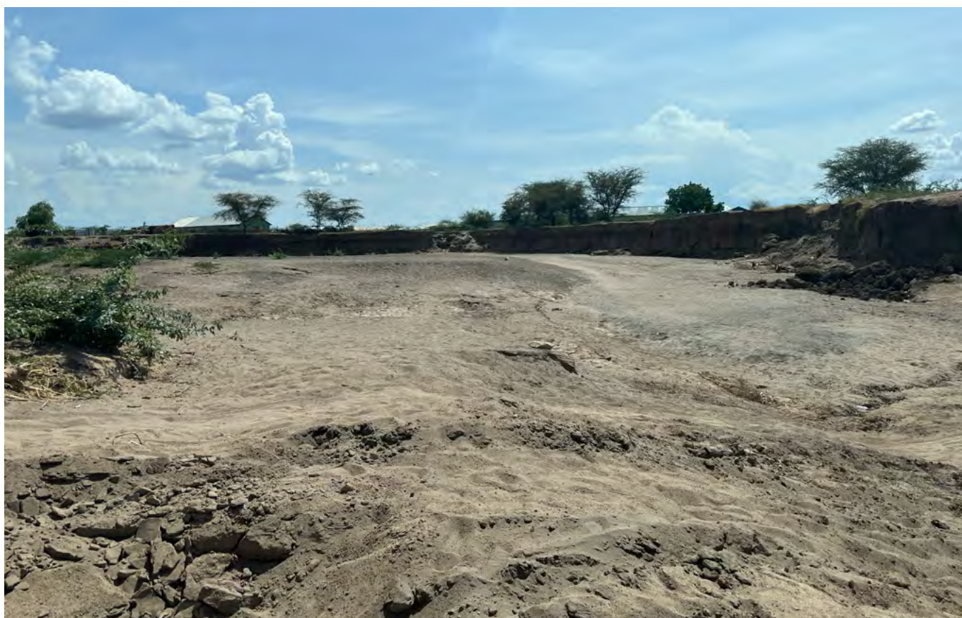
Fig. 40: Significant Erosion Along the Banks of the Lagga Between Kakuma Camps 1 and 2 (UN-Habitat, 2023)
