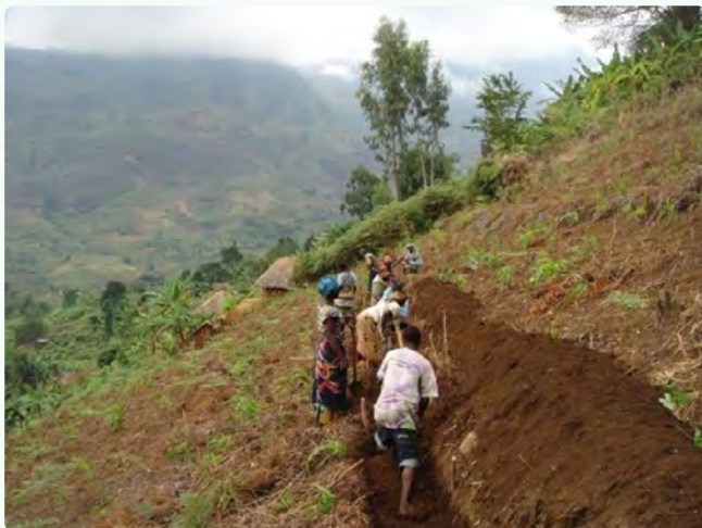
Figure 206 Farmers excavating Fanya Juu terraces to reduce run off and improve crop production 321
