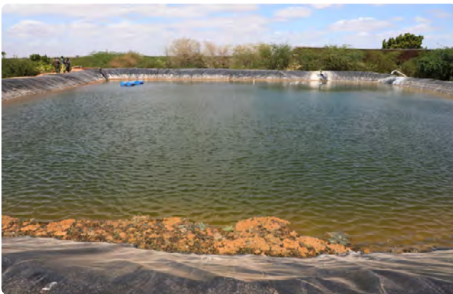
Figure 174 A lined water pan in Dadaab, Garissa County, Kenya
