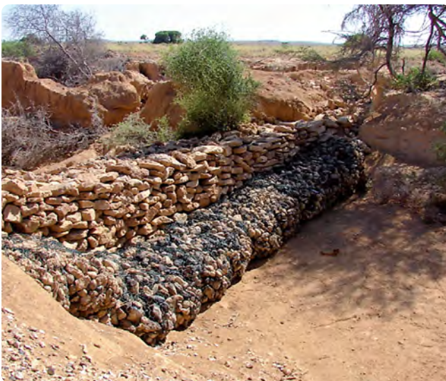
Figure 35 Loose stone dam in East Africa to stop the gully erosion 53
