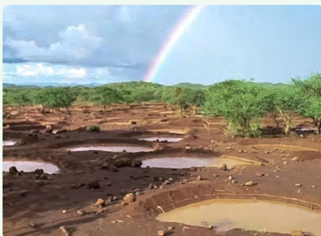
Figure 78 Bunds implemented by Justdiggit in Kuku, Kenya
