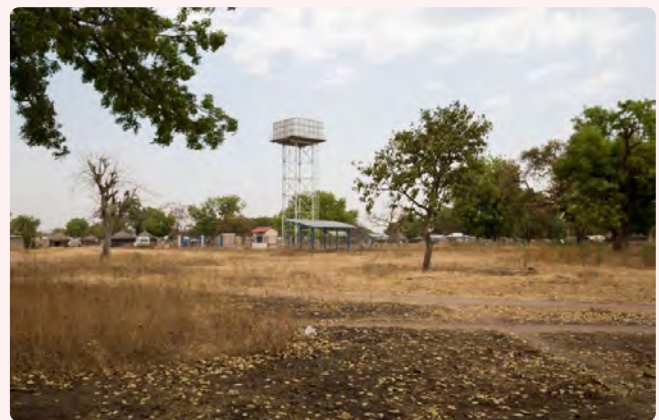
Figure 192 Solar-powered system in Akauch water yard in Rumbek City, South Sudan
