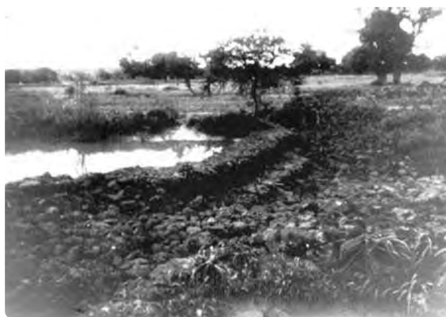
Figure 44 Permeable rock dam spillway 65
