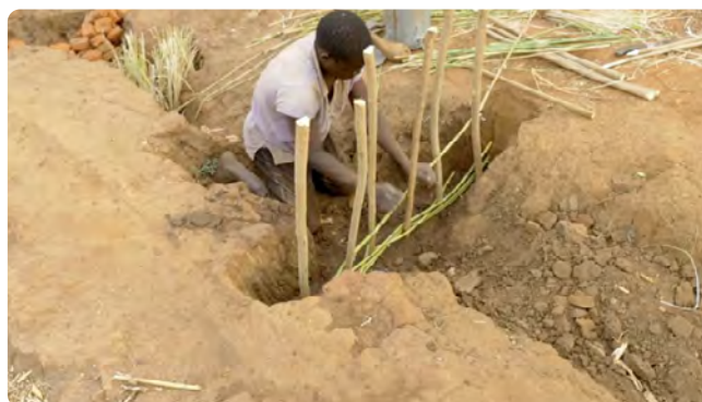
Figure 38 An example of a brushwood check dam under construction 59
