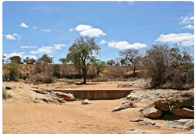
Figure 149 A Sand Storage Dam in the Kiindu river near Kitui, Kenya (2005) 232
