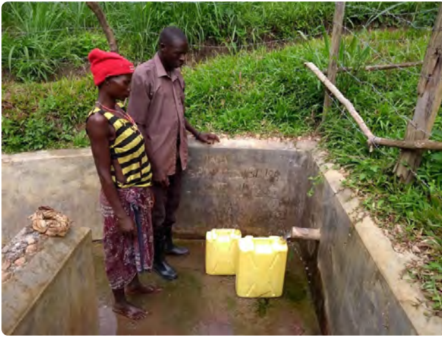
Figure 198 A protected spring for the Abangi-Ndende Community in Uganda 309
