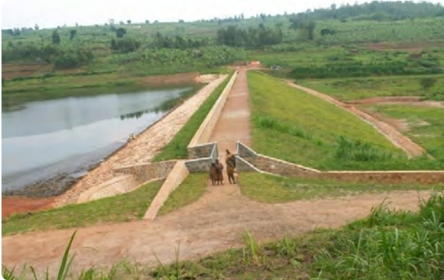
Figure 163 A small earth dam in Kenya 251
