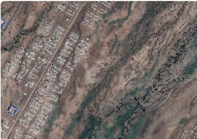
Figure 140 Trapezoidal Bunds along intermittent rivers as viewed from above in Kalobeyei Settlement, Kenya
