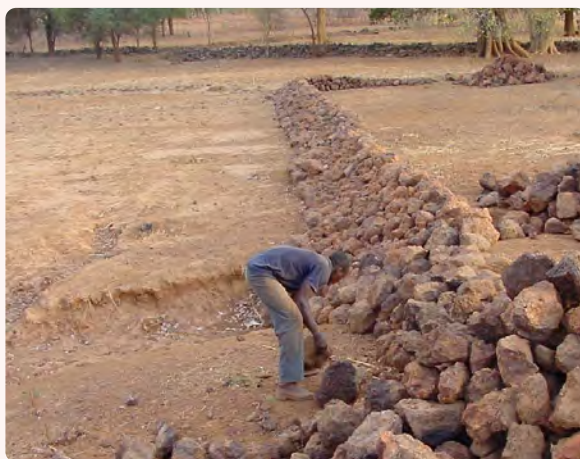
Figure 130 Constructing stone lines 202
