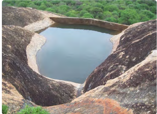
Figure 168 Gravity Wall and Rock Catchment 258
