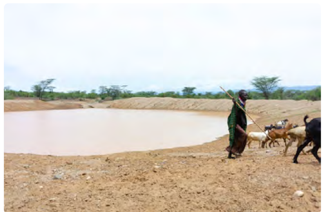
Figure 178 A water pan in Kalobeyei Town supplied by nearby river
