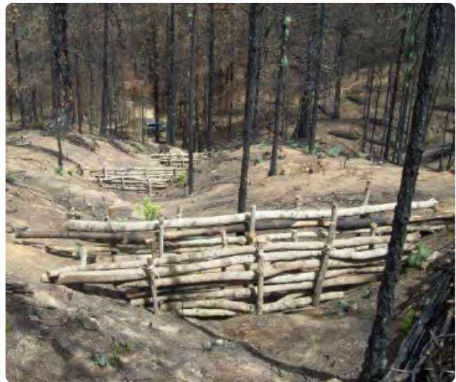
Figure 36 An example of a log check dam 54
