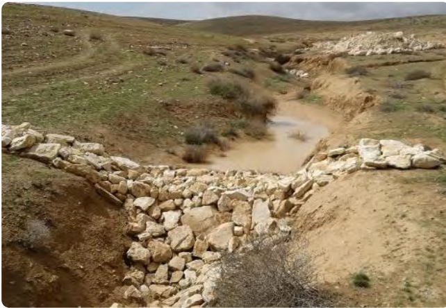
Figure 34 Rock gully plug near Amman, Jordan after rainfall event in 2018 52
