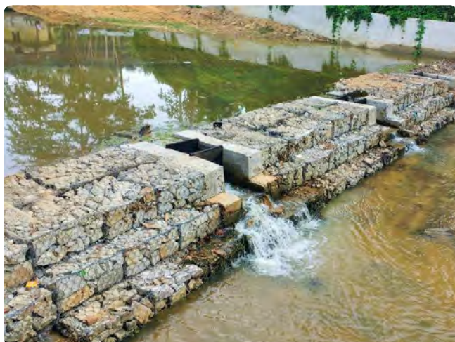
Figure 37 An example of a gabion check dam 58
