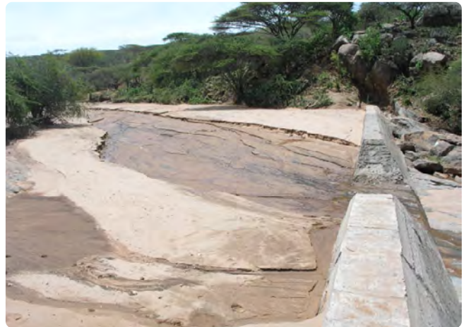
Figure 148 Sand Dam Construction at Kijabe, Kenya 231
