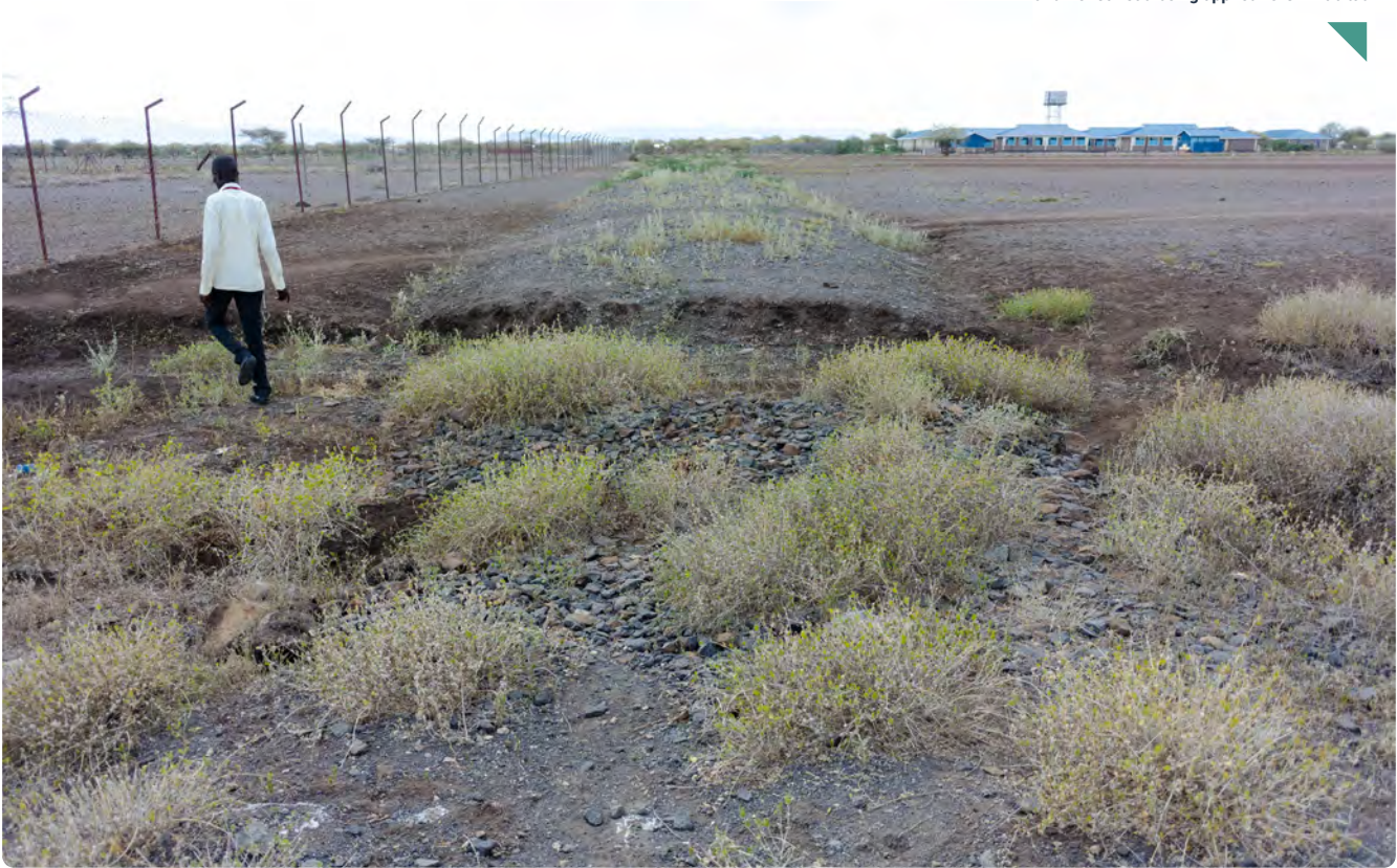
One of the smaller laggas in Kalobeyei Settlement and Donou road being applied. © UN-Habitat
