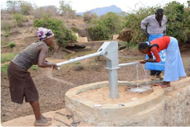
Figure 194 The Water Project: Sand Dams in Kenya, Dug Well and Hand Pump 297
