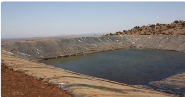
Figure 185 Lagoon Lining 276
