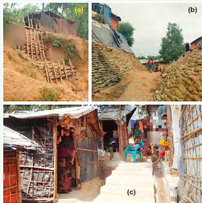
Figure 121 Ongoing site development works
