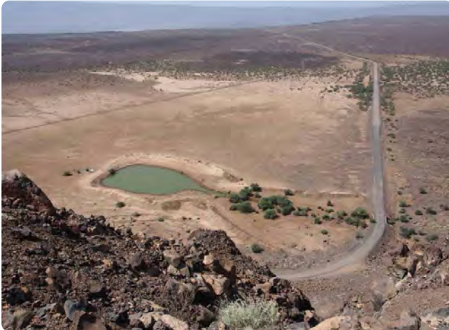
Figure 21 Example of an embankment pond fed by a road culvert 32
