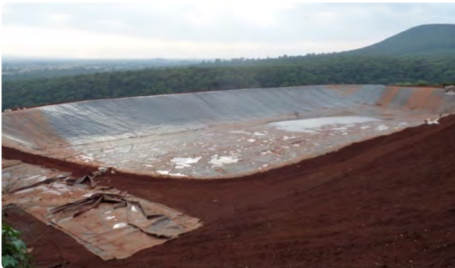
Figure 184 Lagoon Under Construction 275
