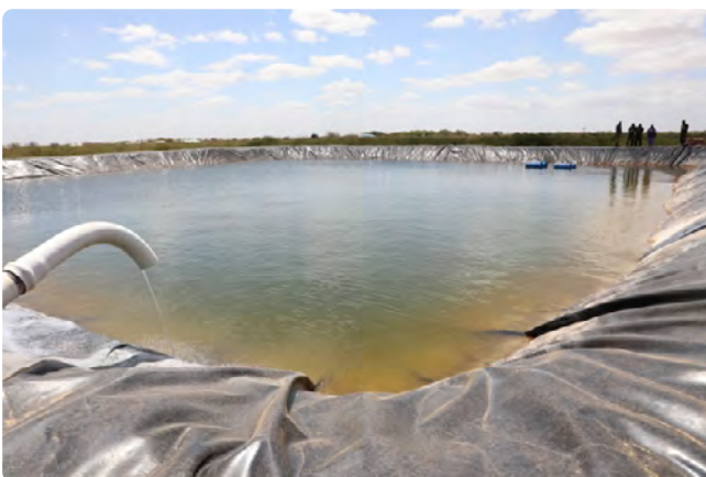
Figure 175 A lined water pan in Dadaab, Garissa County, Kenya
