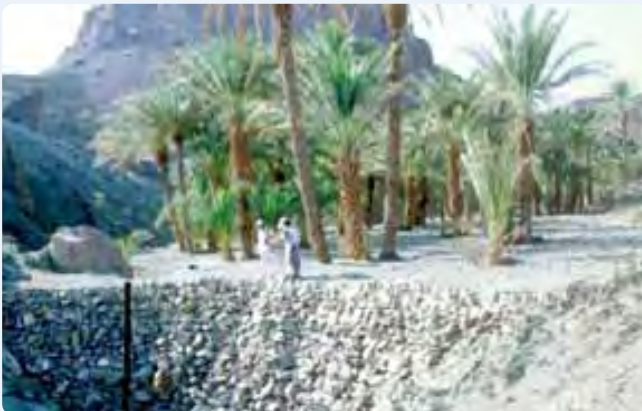
Figure 19 Darband, a spate irrigation system in Baluchestān, southeast Iran 16
