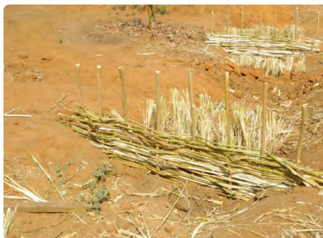
Figure 39 An example of a brushwood check dam 60
