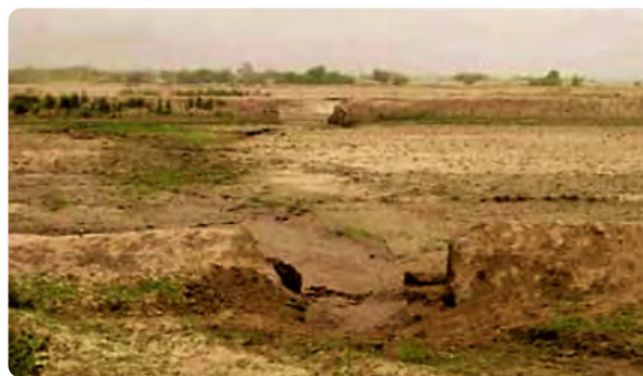
Figure 13 A field-to-field distribution in Eritrea; cuts on the bunds allow water to irrigate the next field 3
