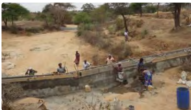
Figure 156 One of the dams under construction 242
