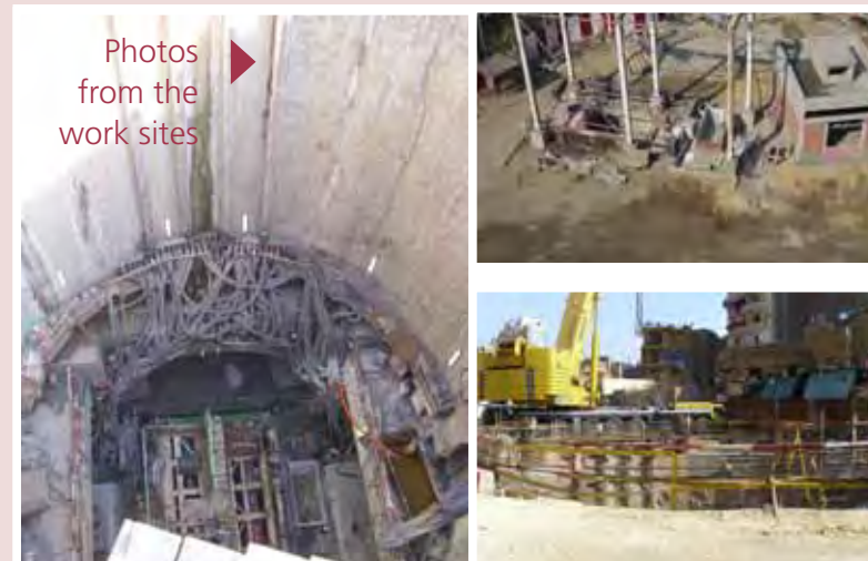
Construction works of the third metro line
