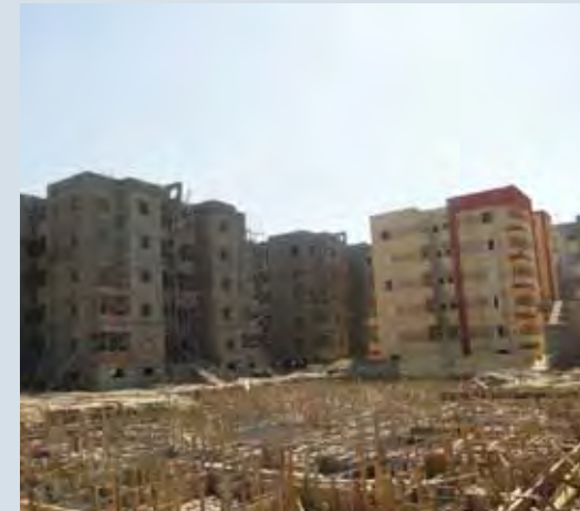
Images showing progress in project constructions
