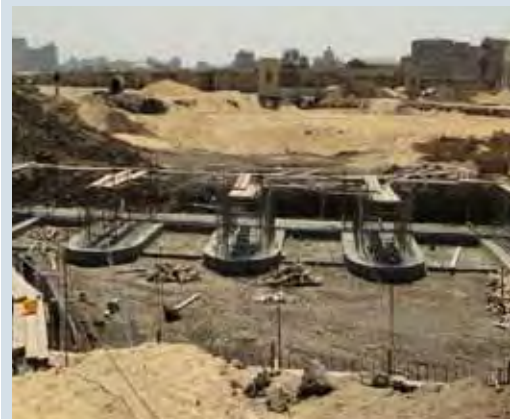
Images showing progress in project constructions
