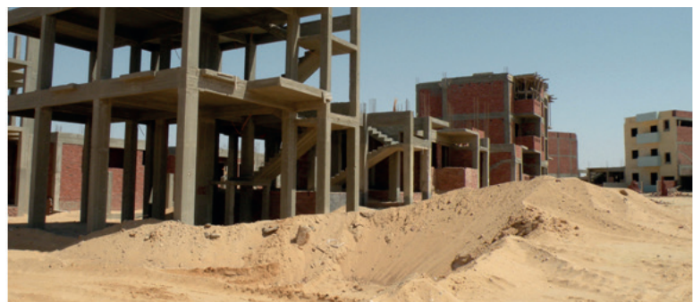
Figure 11.3 Formal private housing under construction, New Cairo, 2009. Photo by D. Sims.
