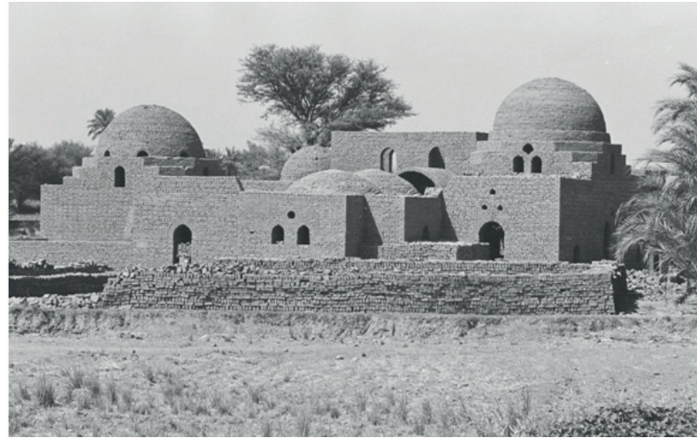
Figure 11.7 Rare example of mud brick residential construction, Al Bairat, Luxor Governorate, 1982. Photo D. Sims
