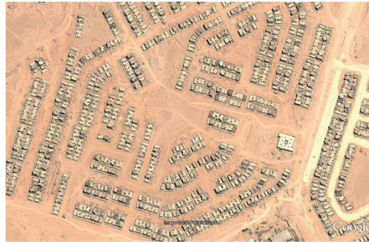
Figure 7.5 Low density neighborhood layout, Ibni Beita sites and services scheme, Sixth of October, July 2013. No inhabitants yet. Google Earth @ 2014, Digital Globe @ 2014.
