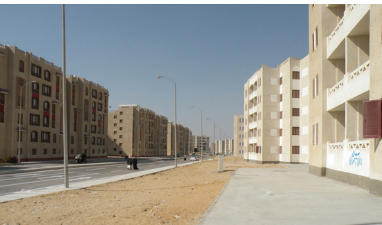
Figure 4.5 NHP tamlik units (each 63 m 2 ) in 6 October City, 2010. Photo: David Sims
