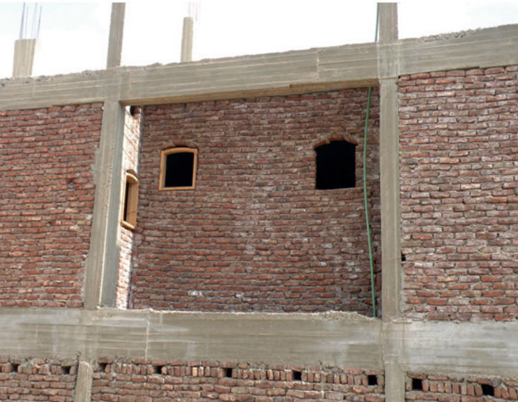
Figure 11.6 Example of red brick infill in informal construction. Note the small light well provided. Al Bairat, Luxor Governorate, 2015. Photo by D. Sims
