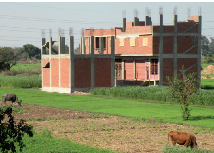
Figure 7.9 Piecemeal informal housing construction on converted agricultural land, Waraq, Giza, 2011. Photo by D. Sims
