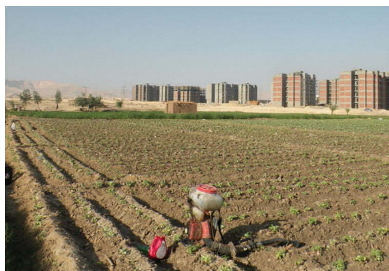
Figure 4.11 Remote governorate social housing blocks under construction on Western Desert fringe. Armant, Luxor Governorate, January 2014. Photo: D. Sims
