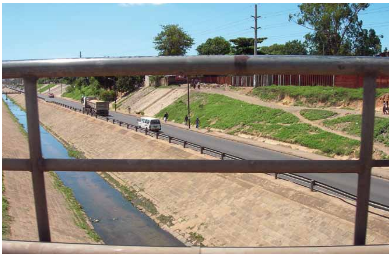
Adapting to climate change. Improved storm water drainage in Maputo ©UN-HABITAT/B. Oballa
