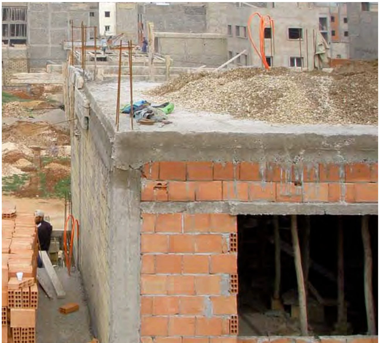
Construction Site Bidonville © ETH Studio Basel
