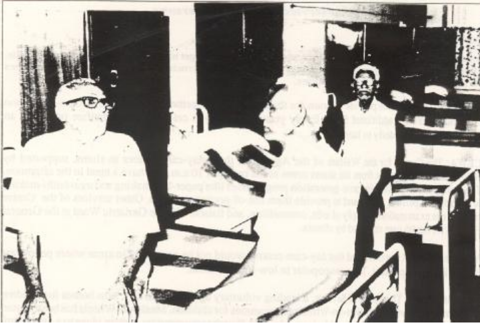
Figure 9. Dormitory at Home for the Aged, Little Sisters of the Poor
