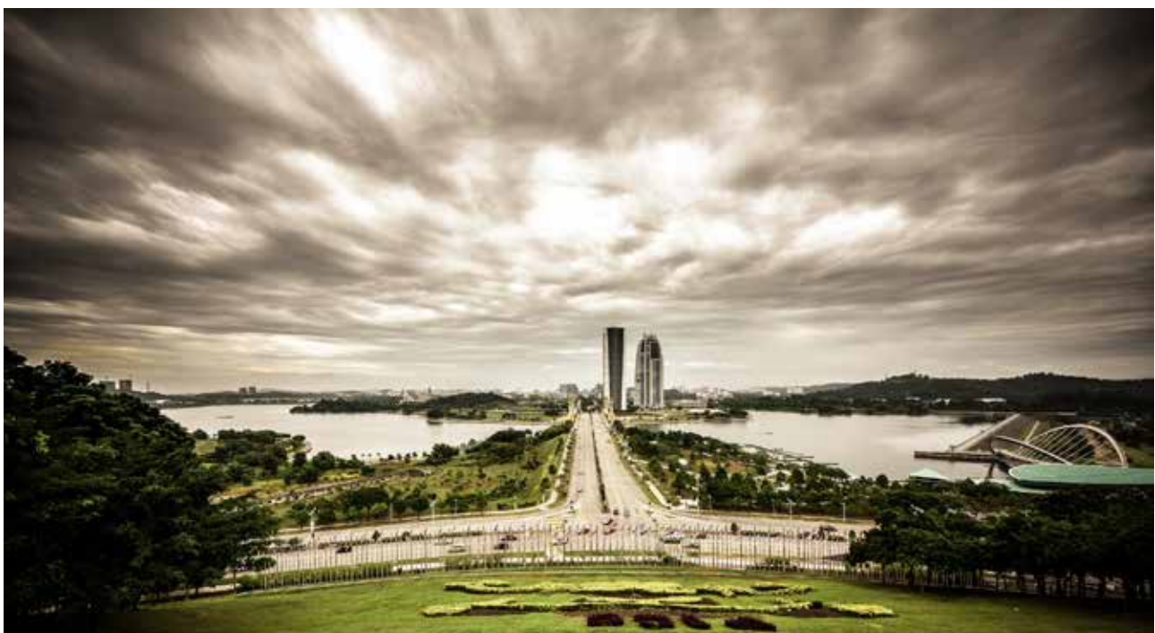
Putrajaya International Convention Centre © Flickr/taufuuu
