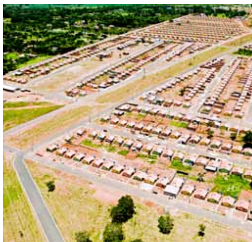
Roadways for new housing, Uberlandia, Brazil © UN-Habitat/Alessandro Scotti
