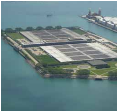
Water treatment plant in Chicago, USA © Flickr/Neal Jennings/Sweet one
