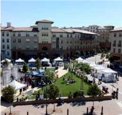
A mixed-use development with public space near a transport node in Walnut Creek, California © Sam Newberg
