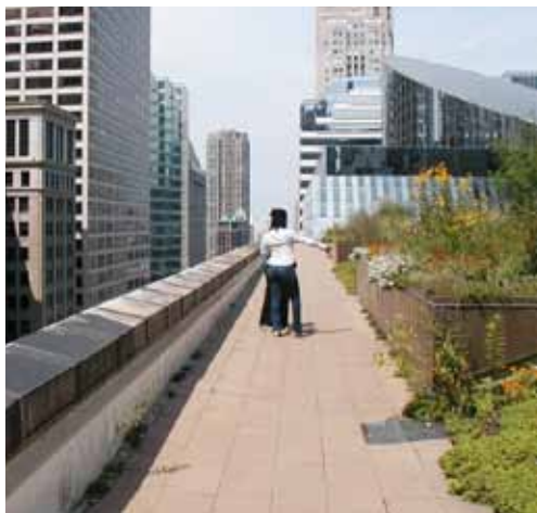
Chicago City Hall Green Roof, USA © Flickr/TouringCyclist
