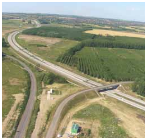
Infrastructure is a significant enabler of urban growth, Budapest, Hungary © Akil Sokoli
