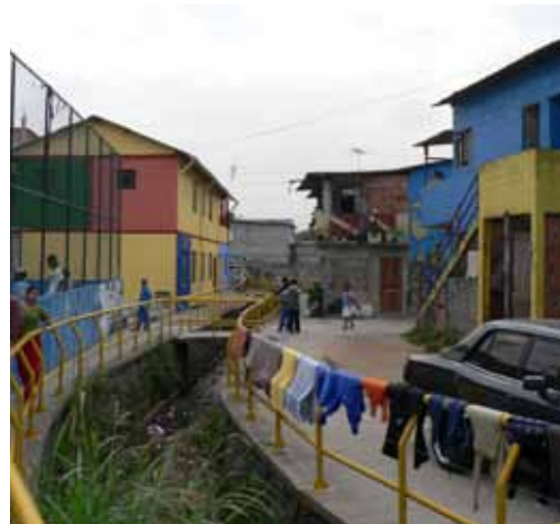
Drainage infrastructure in Jardim Iporanga, Sao Paulo, Brazil © Affordable Housing Institute
