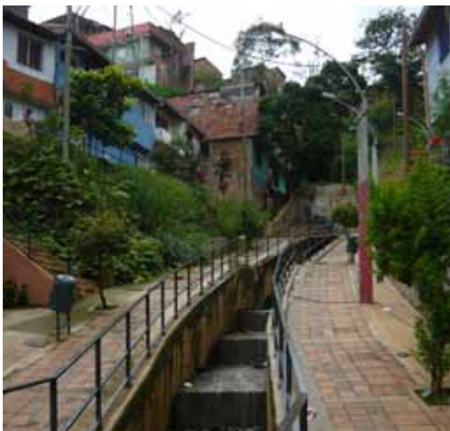
Drainage infrastructure greatly improves the conditions of sloping areas in Medellín, Colombia © UN-Habitat/Laura Petrella
