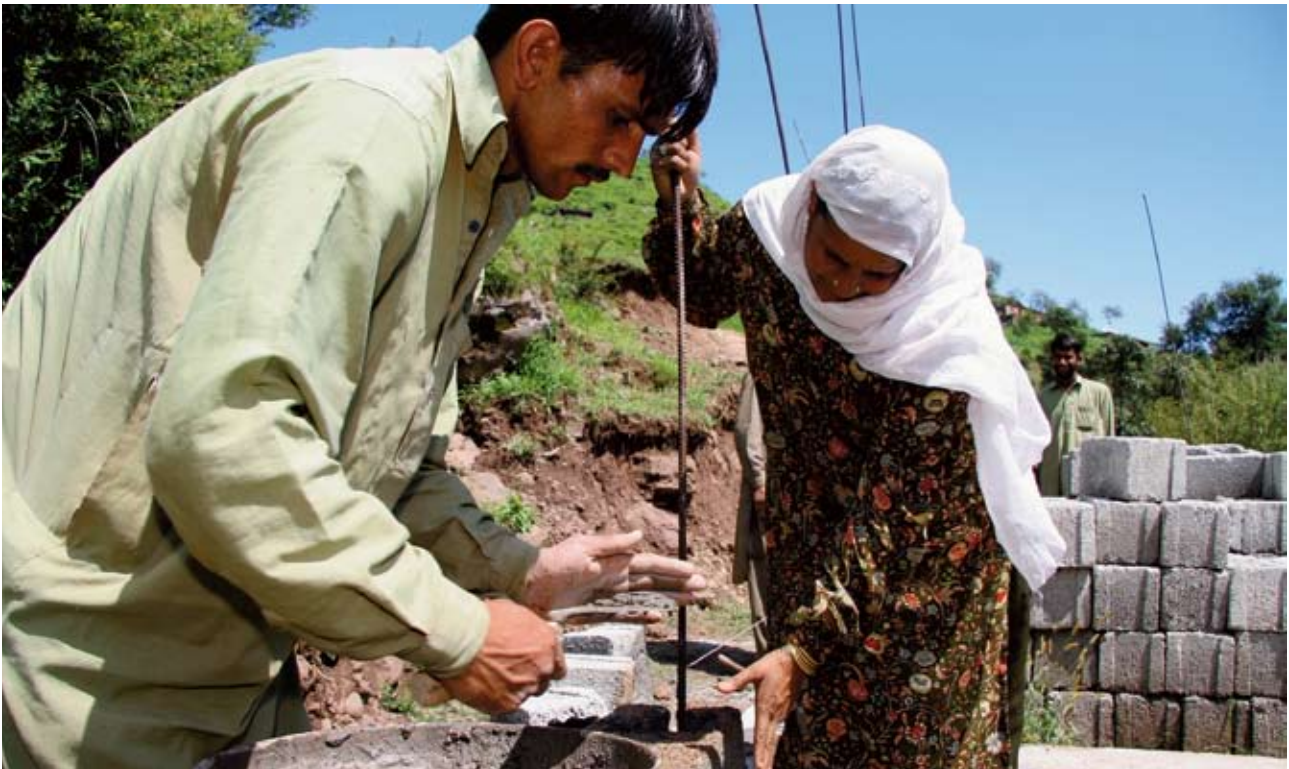
Widow supervising reconstruction of her new house, Kashmir © V.Wijaya / UN-HABITAT
