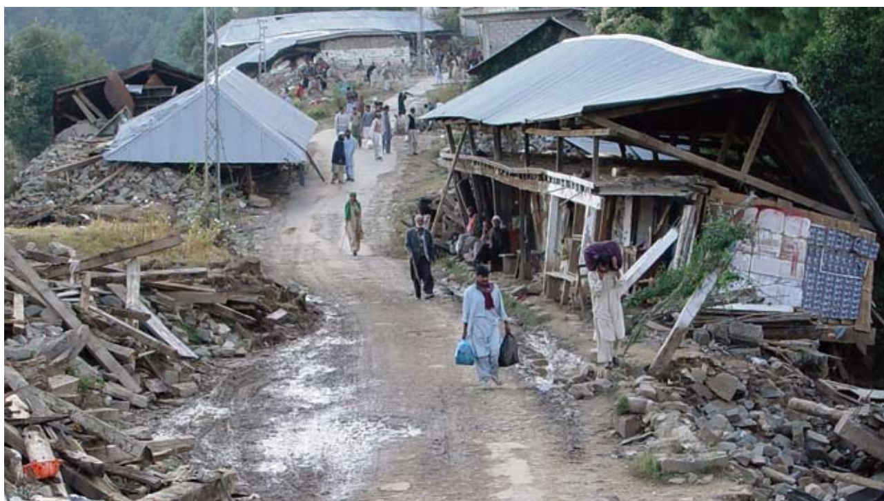
Destruction caused by the Kashmir earthquake 2005 © UN-HABITAT / M.Stephenson
