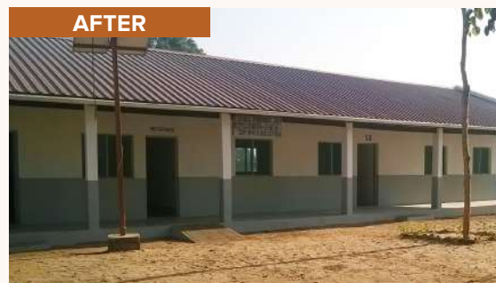
UN-Habitat cyclone resilient design used to rebuild schools in Nampula District, Mozambique ©UN-Habitat
