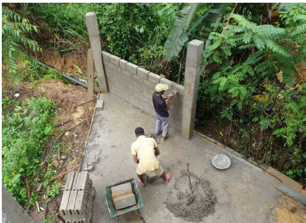
Building a concrete retaining wall in Sri Lanka © Shutterstock
