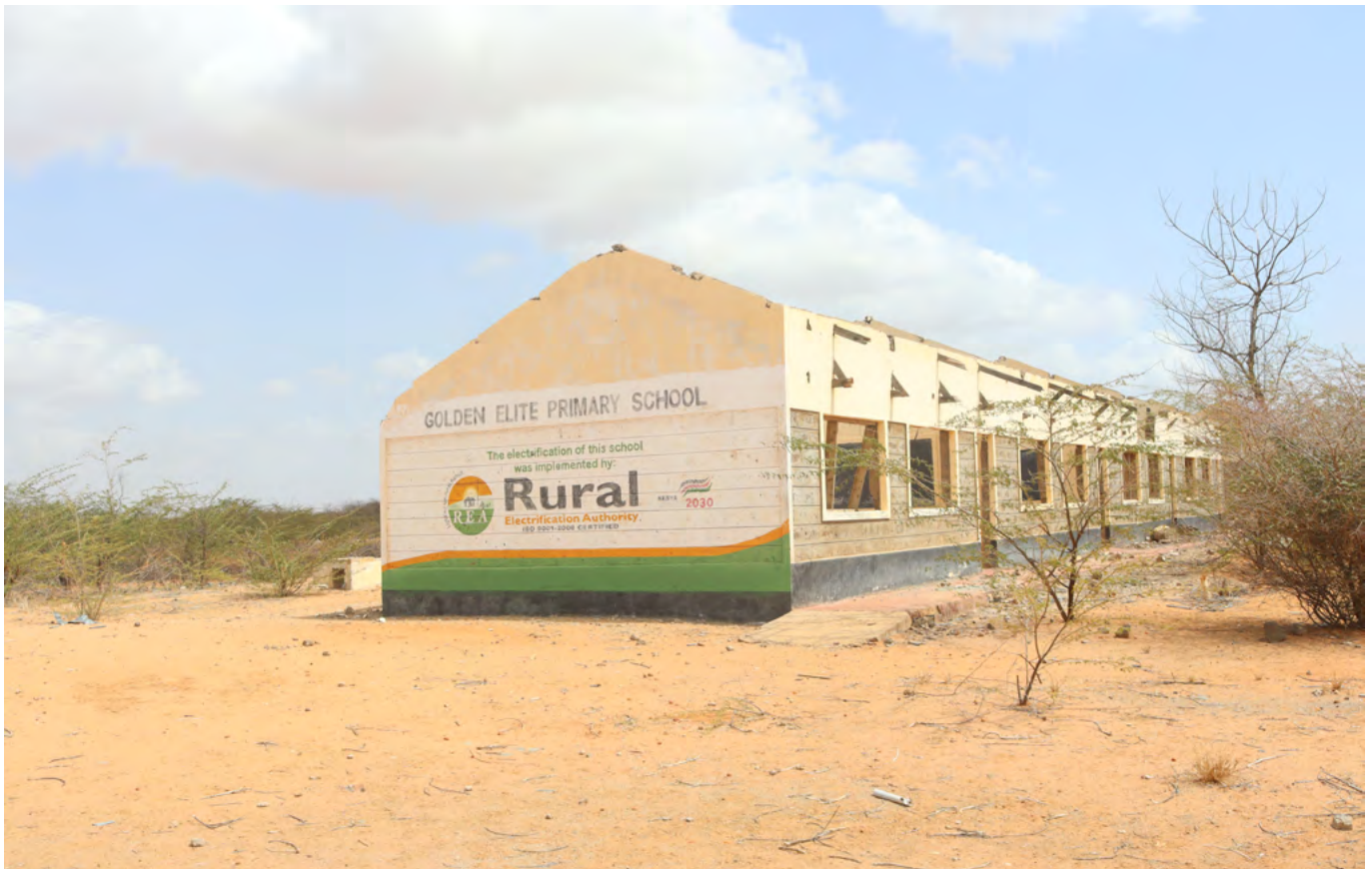
Fig. 31: An Example of a Dilapidated Closed School Structure in Kambioos (UN-Habitat, 2022)
