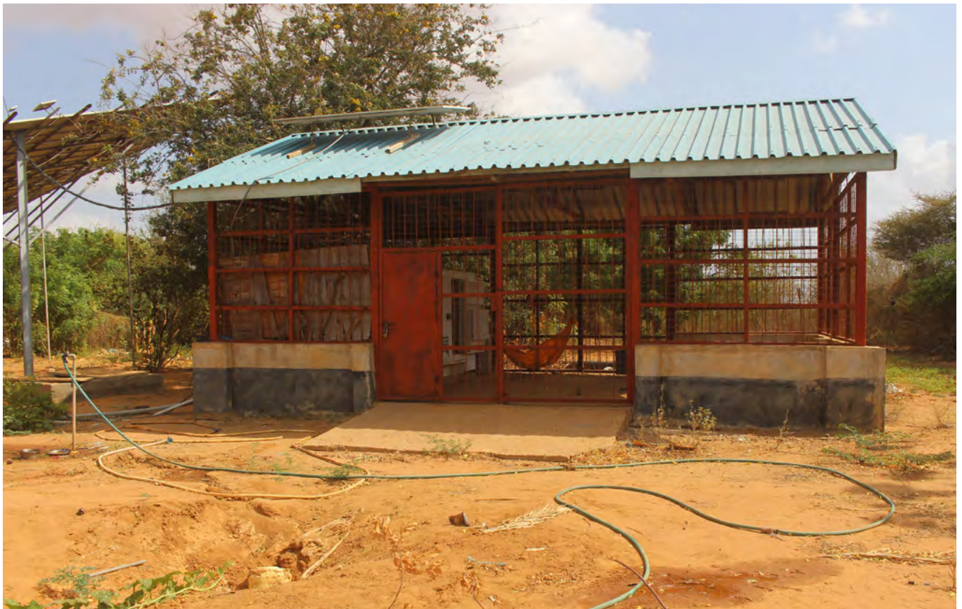
Fig. 62: Water Pumping Unit, Ifo 2 Camp (UN-Habitat, 2022)
