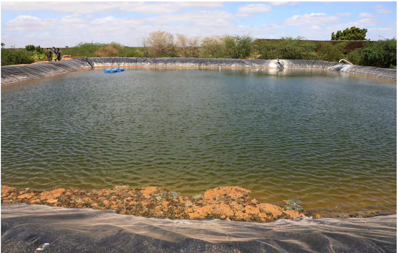
Fig. 53: A Water Pan In Ifo 2 Camp Serving Orchard Farms Near Mwangaza Primary School (UN-Habitat, 2022)
