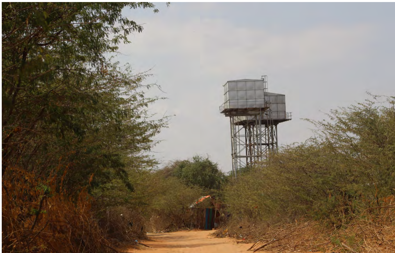
Fig. 61: Water Pumping Unit, Ifo 2 Camp (UN-Habitat, 2022)
