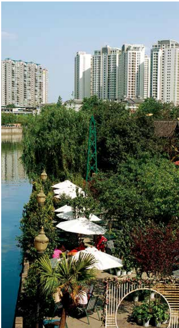
▲ 成都（四川省，中国中部），府南河的综合整治工程需全部拆除原河岸贫民住宅并原地安置原居民。 In Chengdu (Sichuan, central China), comprehensive revitalization of the rivers Fu and Nan has entailed the removal and subsequent on-the-spot relocation of those living in the riverside slums. ©Fenghui/Shutterstock
